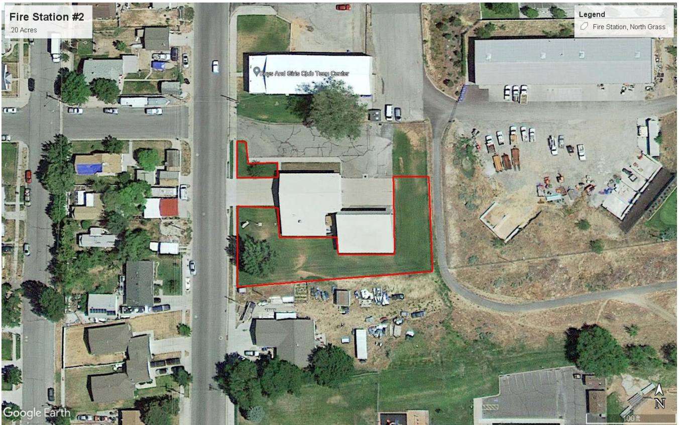
Location No. 11 - Fire Station No. 2
